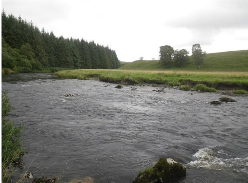
Figure 12: Site SRWF7, looking upstream from the right bankside
